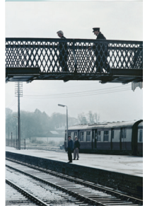
Railway overbridge, Antrim train station, Northern Ireland, 1970s
